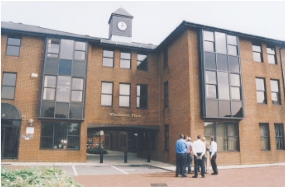
The exterior of Parkegate Engineering's offices at Winchester Place, Poole
